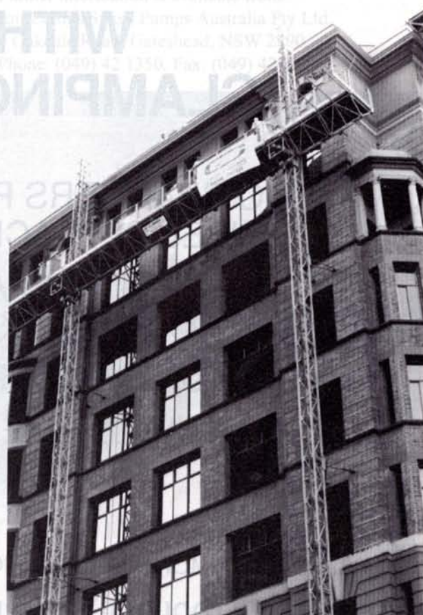
Hi-Climber in use on heritage building, Daking House, where an ornate concrete hood was cut back and replaced.
